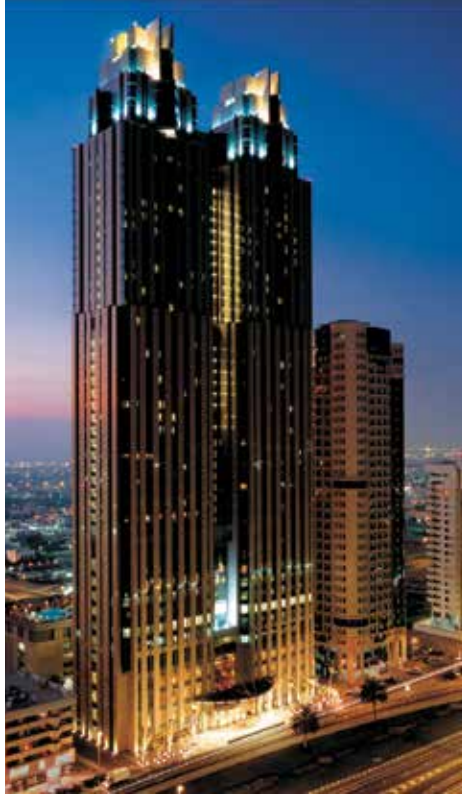
Exterior of Shangri-La hotel / DUBAI
