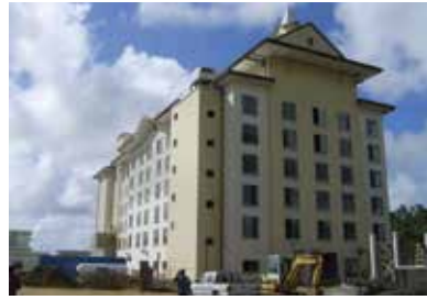
Marriott Courtyard hotel Paramaribo / SURINAM
